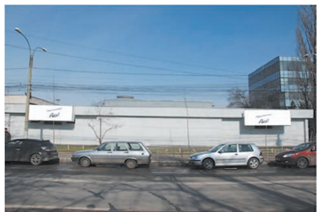
BANNER DISPLAY ON ROMEXPO HEADQUARTER FACADE
